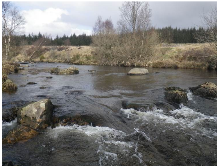
Figure 35: Large boulders have been artificially placed across the river
